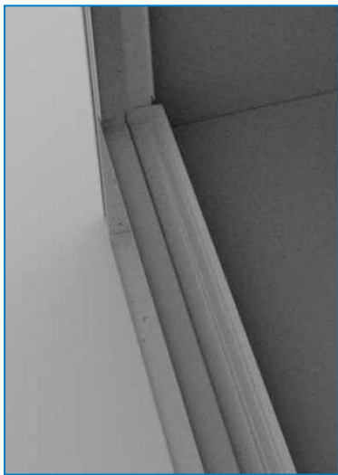
Water collection gutter
