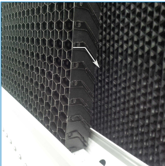
Orientation of the combined inlet shield
