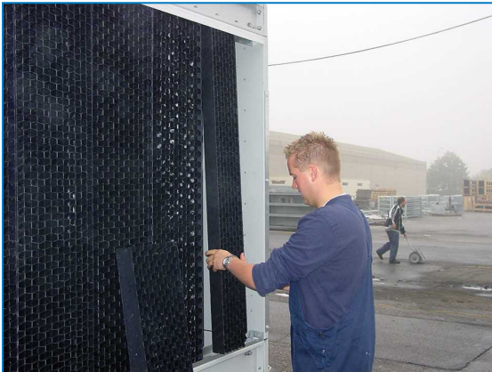
Remove combined inlet shields
